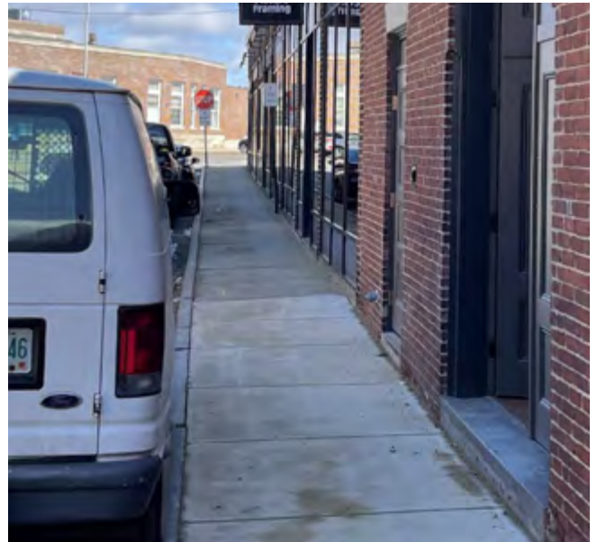
6" LIFT FROM SIDEWALK TO LOAD-IN LEVEL
